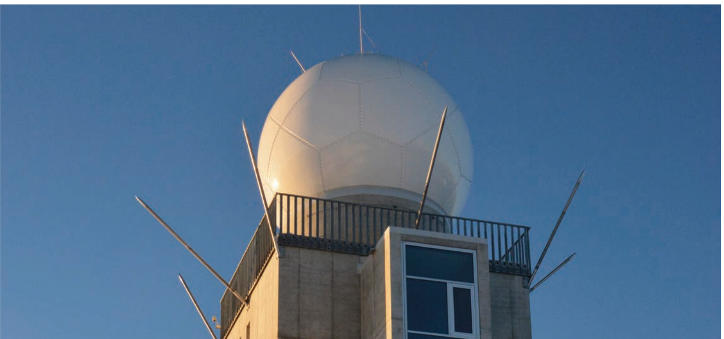
Weather radar system
