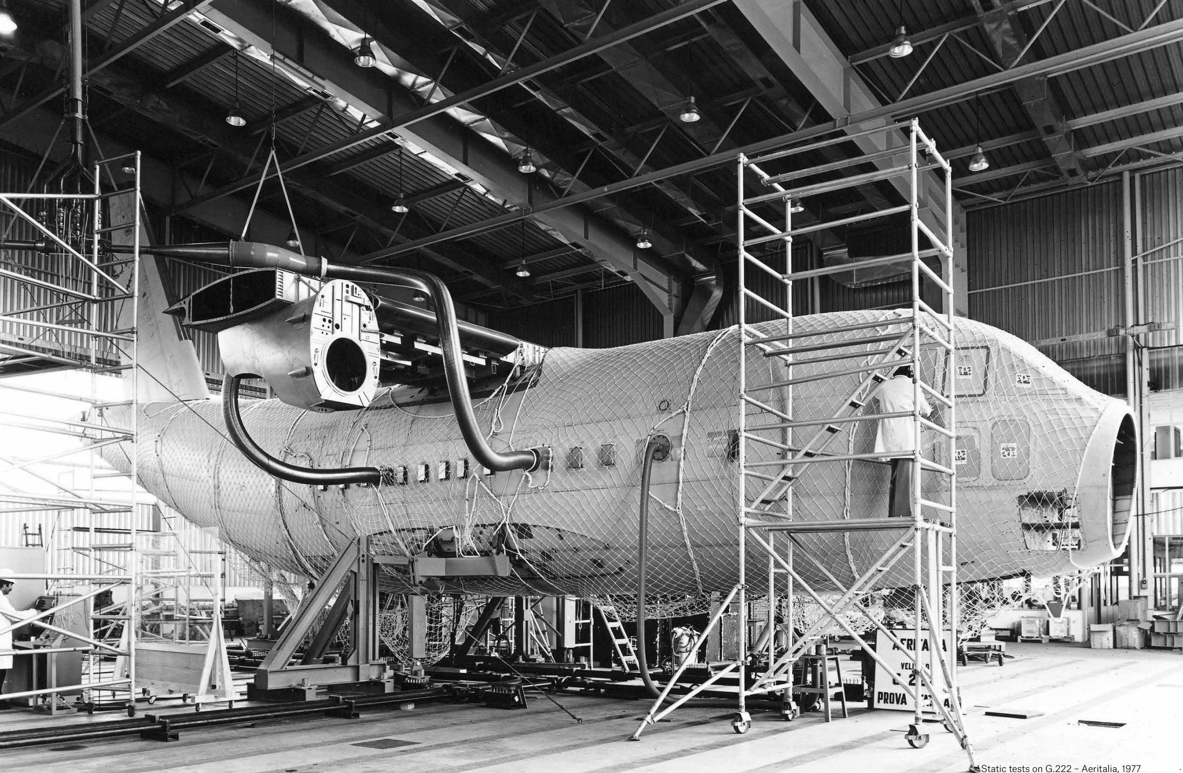
Static tests on G.222 - Aeritalia, 1977
